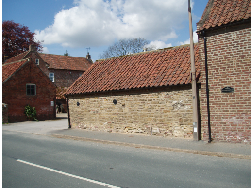
One of the few remaining examples of Wolds stone walling, at Manor Farm
