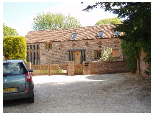
Rectory Barn – An excellent example of how to convert a redundant agricultural building into a 21 st century dwelling, without losing its character.
